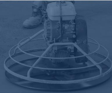
**FIBERMESH®** synthetic fiber, **ENDURO® 600**, **NOVOMESH®** fiber blend and **NOVOCON®** steel fiber reinforced concrete (FRC) slabs can achieve the same high-quality finishes as plain concrete. Whatever the required finish, satisfactory results can be obtained with synthetic and steel fibers if proper placement and finishing techniques are followed. As always, timing and technique are important when finishing fiber reinforced concrete slabs.
